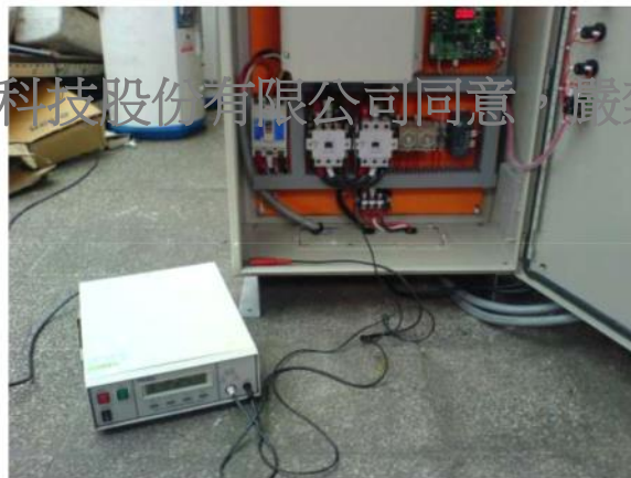
Insulation resistance test
